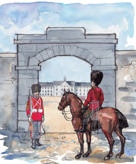
Entrance arch of West Barracks [34]
